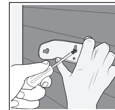
2. Line the mounting bracket up with the holes and drill the screws into the wall with a screwdriver or drill.
